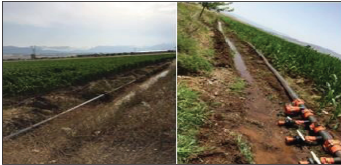
Figure 11. Overview of the closed pipe system
